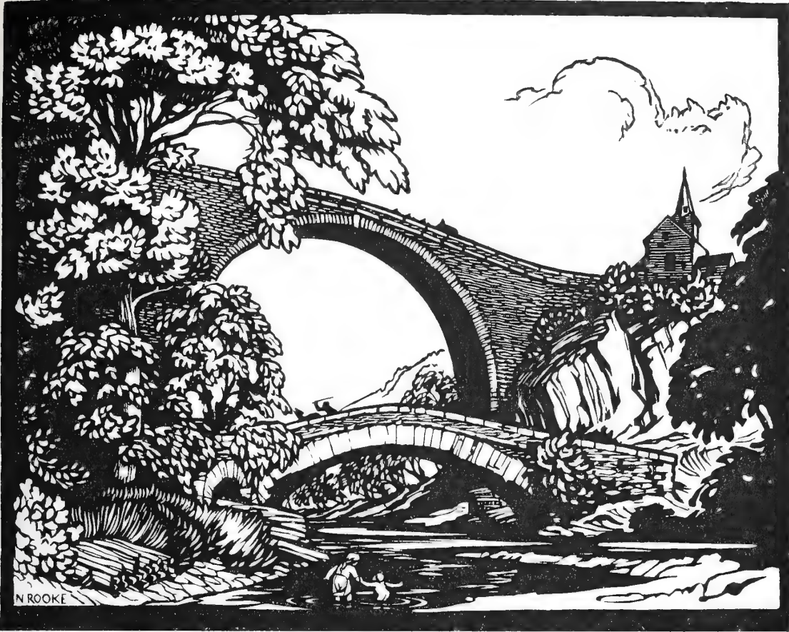
“THE TWO BRIDGES”
